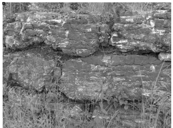
Fly-ash blocks at Jacksdale wharf
