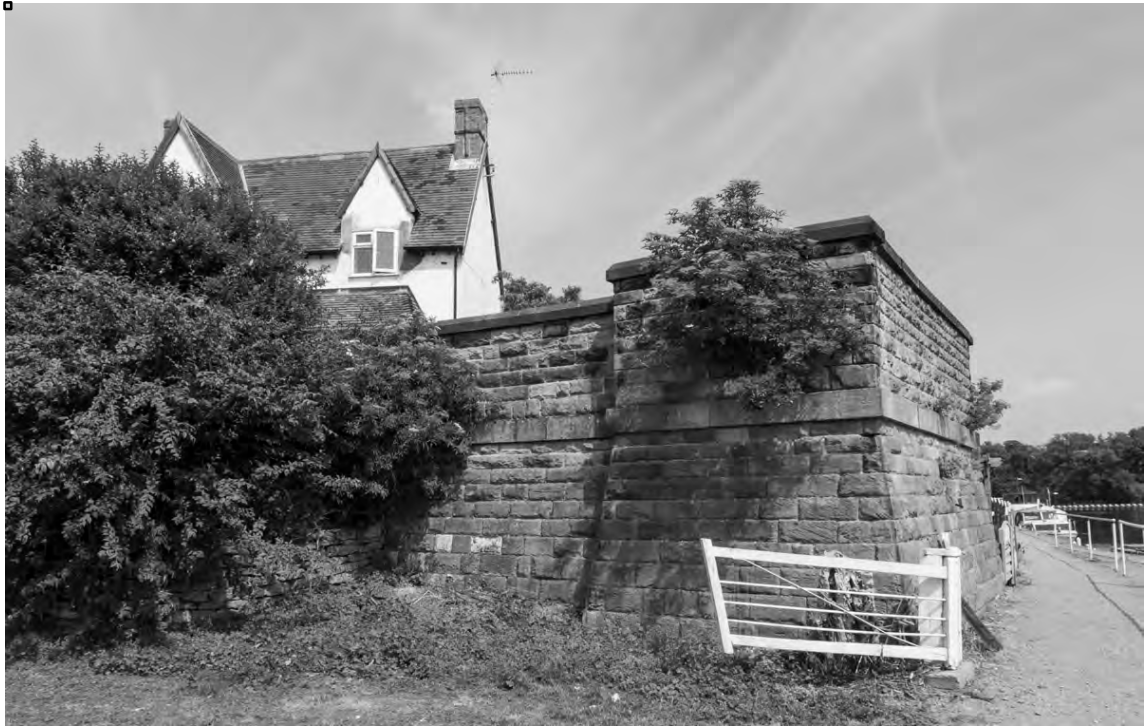
Above: The old iron bridge abutment on the north bank of the river with the toll house (now a restaurant) seen from the river bank.
